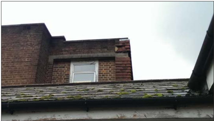
Figure 7: Loose tiles on Cheviot House
