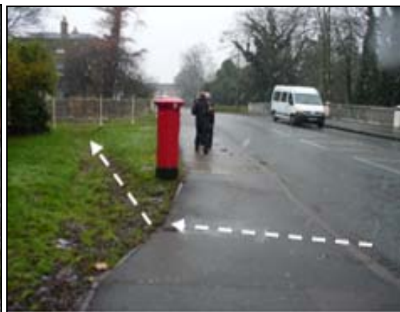
Figure 4-10 Swale at Riverside Close
