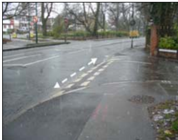
Figure 4-9 Bund at Riverside Close
