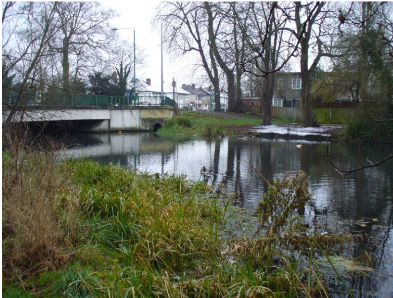
Figure 3-10 Surface water outfall into River Wandle
