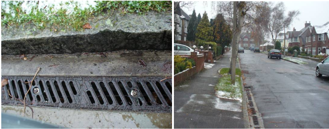
Figure 3-12 Linear Drainage Gullies, Revell Road
