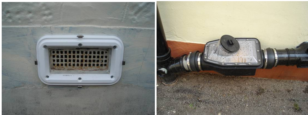
Figure 4-8 Floodguards Property Level Protection; air bricks and non-return valves
