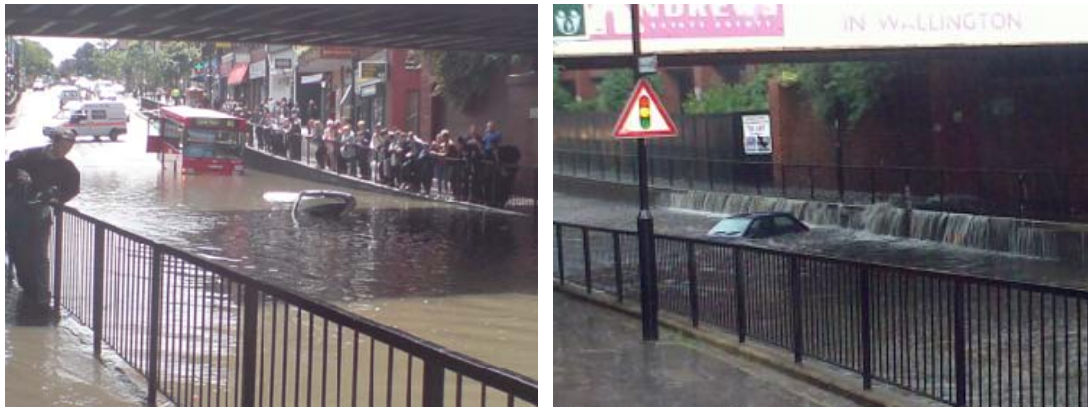
Figure 3-9 Flooding at Wallington Railway Bridge (Source: www.yourlocalguardian.co.uk )
