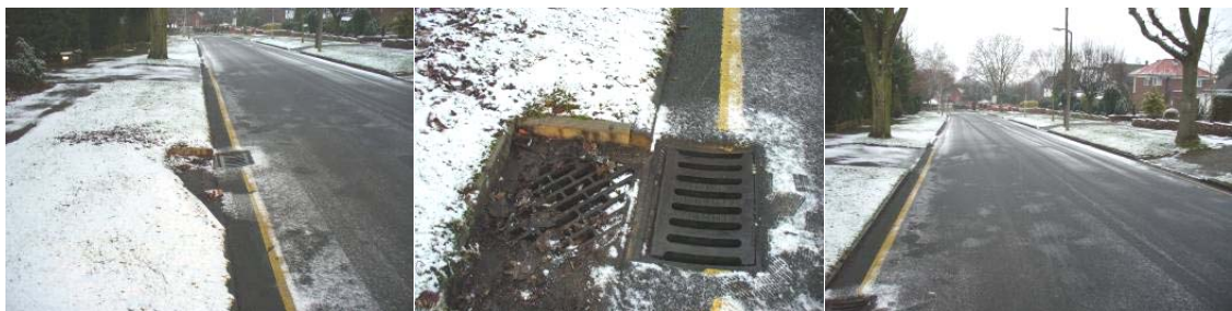
Figure 3-13 Drainage Improvement Works, The Gallop
