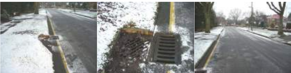
Figure 3-13 Drainage Improvement Works, The Gallop
