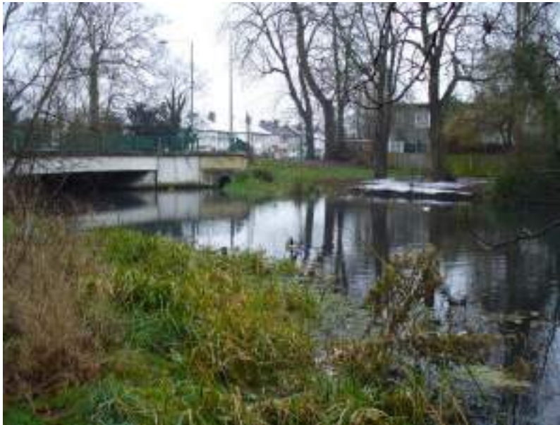
Figure 3-10 Surface water outfall into River Wandle
