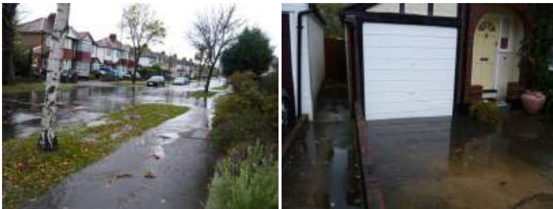
Figure 3-14 Surface water flooding, Church Hill
