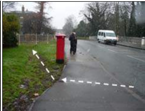
Figure 4-10 Swale at Riverside Close
