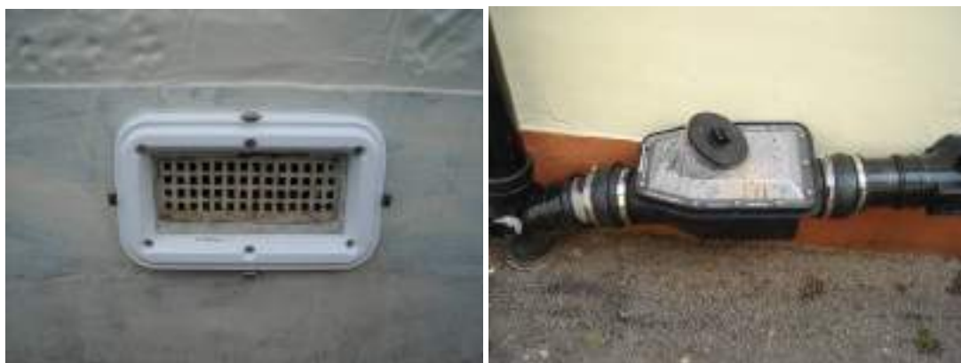
Figure 4-8 Floodguards Property Level Protection; air bricks and non-return valves
