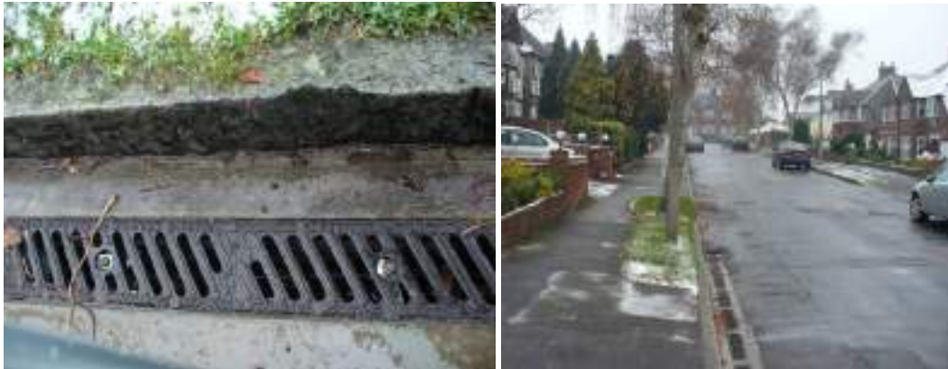
Figure 3-12 Linear Drainage Gullies, Revell Road
