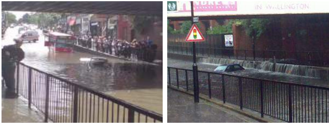
Figure 3-9 Flooding at Wallington Railway Bridge (Source: www.yourlocalguardian.co.uk )
