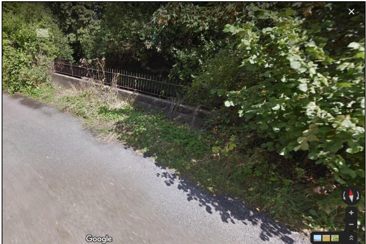
Figure 3.3. EA raised flood wall – adjacent to Watermead Lane (Google Maps, 2020)
