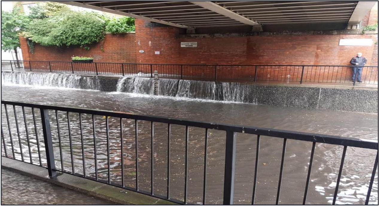
Figure 2-3. Water surcharging from manhole on the footway which resulted in flooding of the highway underneath Wallington Bridge - © Resident, 2017
