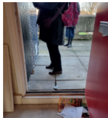
Stepped thresholds: poor accessibility
