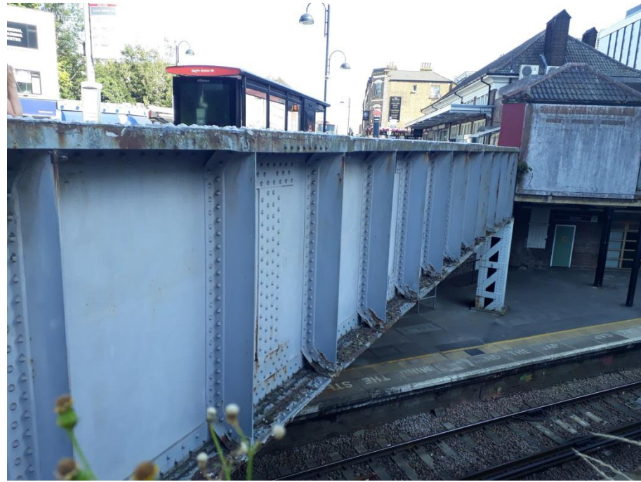
c) Bridge over railway line (Sutton station)
