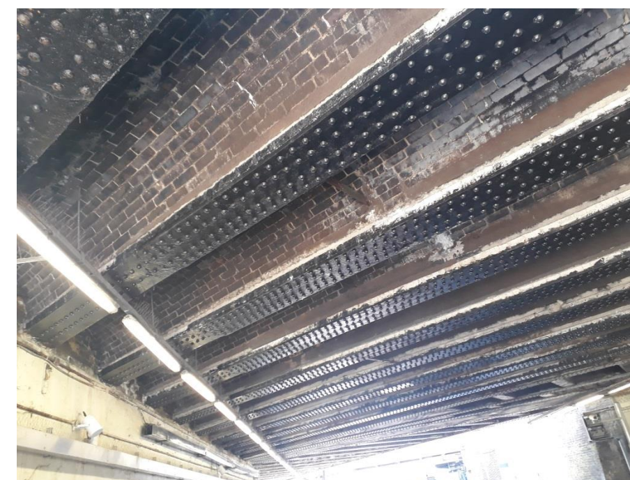
b) Underside of bridge over railway line (Sutton Station)
