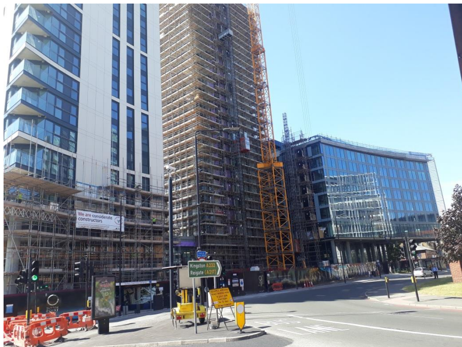
l) South of Sutton Court Road site
