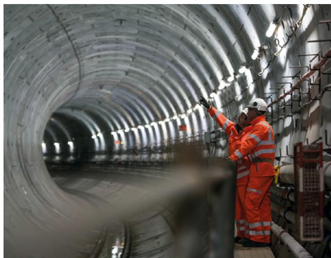
The Tunnel is on track to be in service by 2025. On its own, with an investment of £4.6 billion, it represents the largest and most significant wastewater project since Sir Joseph Bazalgette created London’s sewage system in the 1860s. The Tunnel is 25 kilometres long and up to 75 metres deep, running beneath the river from Acton in West London to Beckton in East London.
