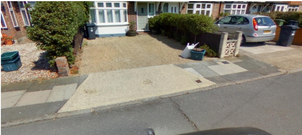
Photo 4: A Shingle (Loose Surface) Hard Standing
