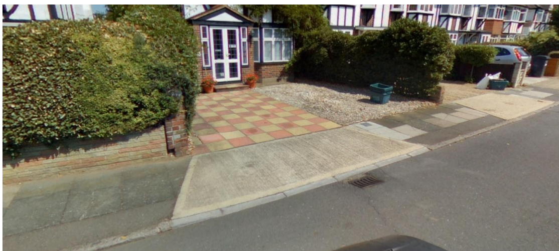
Photo 5: A Permeable Paving Hard Standing
