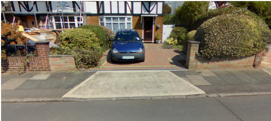
Photo 1: Typical Concrete Vehicle Crossover
